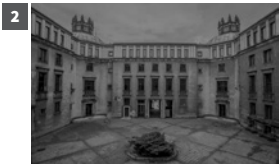
2. Courtyard of the management building, Administrative Centre of the Lenin Steelworks. Photo by Tom Rollauer, courtesy of NCA sp. z o.o.
